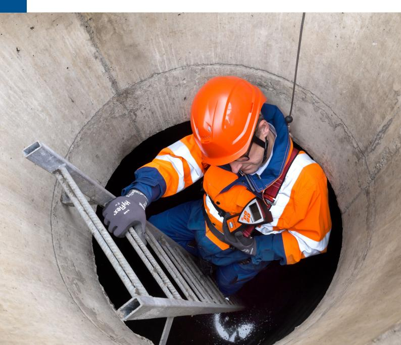
Excessively high concentrations of dangerous gases (e.g. methane, carbon monoxide, hydrogen sulphide) can be harmful to health or even life-threatening.
